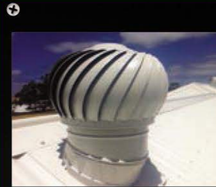
Roof ventilators to keep air fresh
